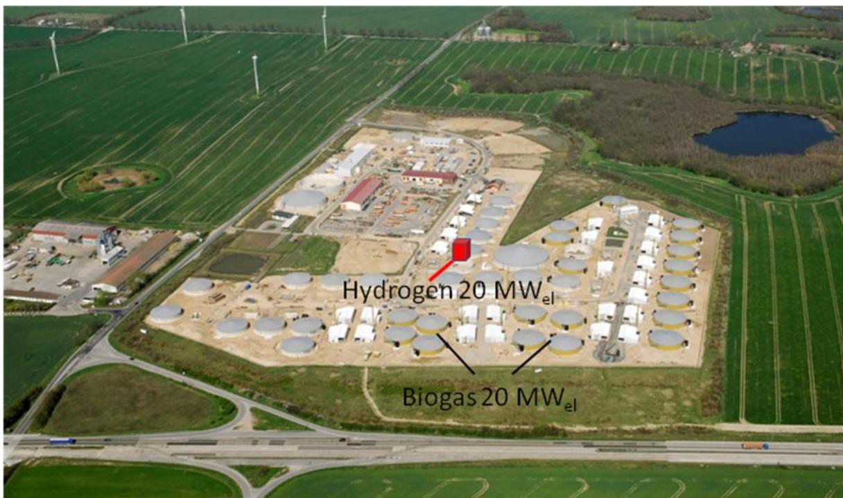
**Fig. 10 Digestive and Chemical Plant Compared**
